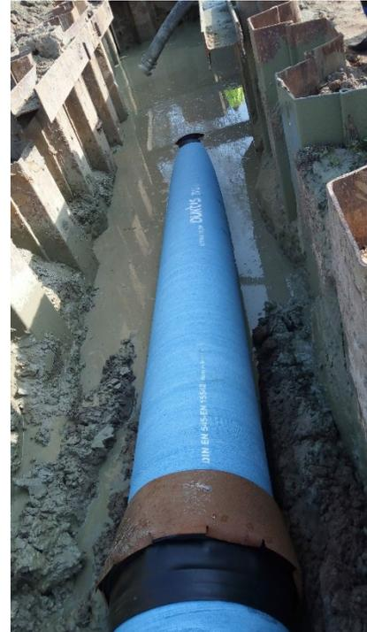
*Performance test of the drill head prior to pulling in the pipe – pulling the pipe into the borehole*
