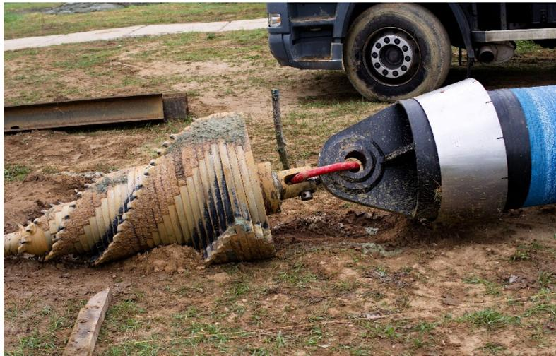
*Connecting the expansion head and 600 mm nominal diameter pulling head*
