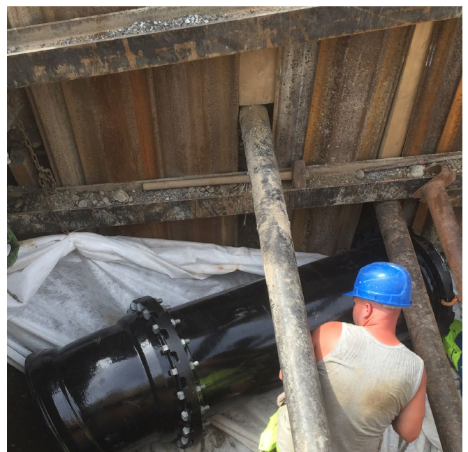
DN 600 ECOPUR installation in a shored trench
