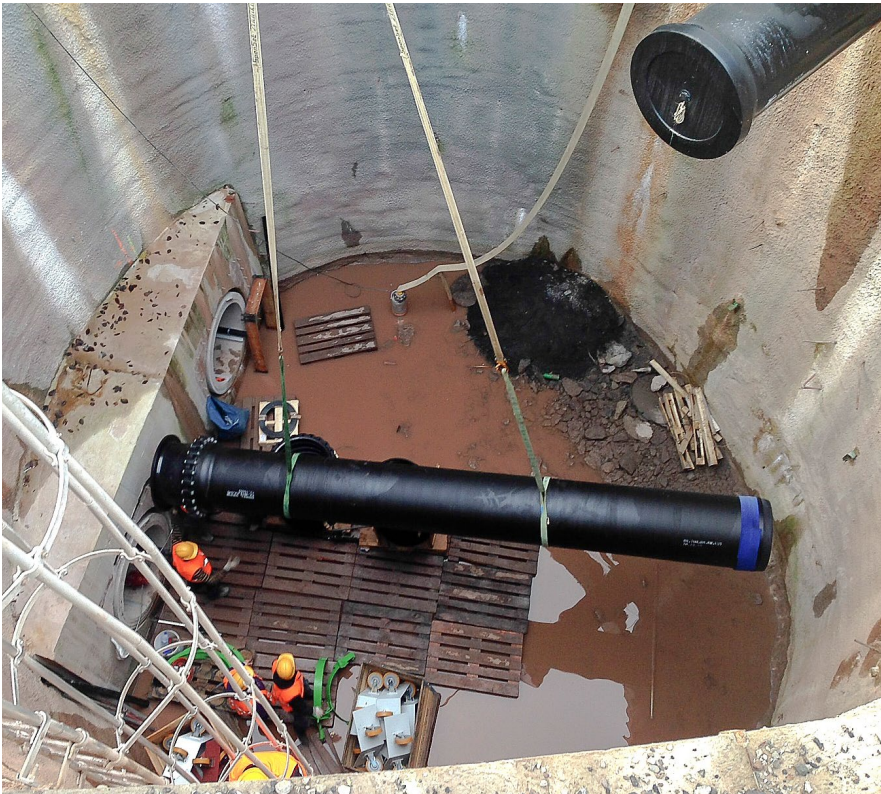
DUCPUR DN 700 double pipeline in a shaft, entry into concrete micro tunnel
