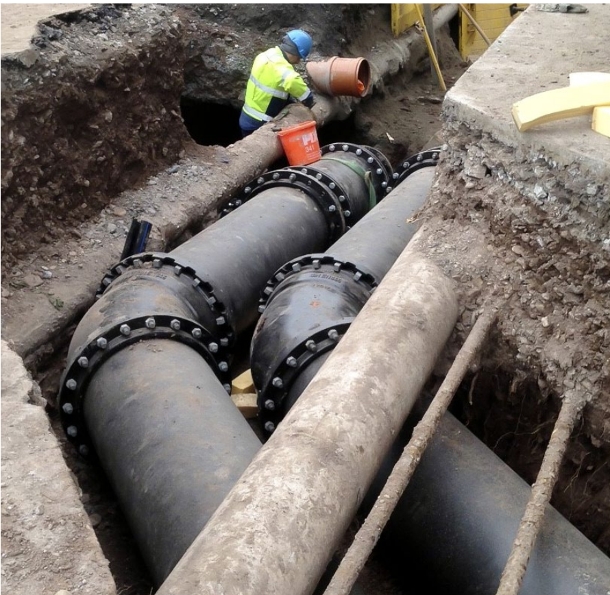
vonRoll DUCPUR, double pipeline with flow and return
